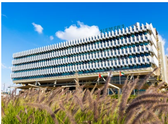
Siemens Energy Building
